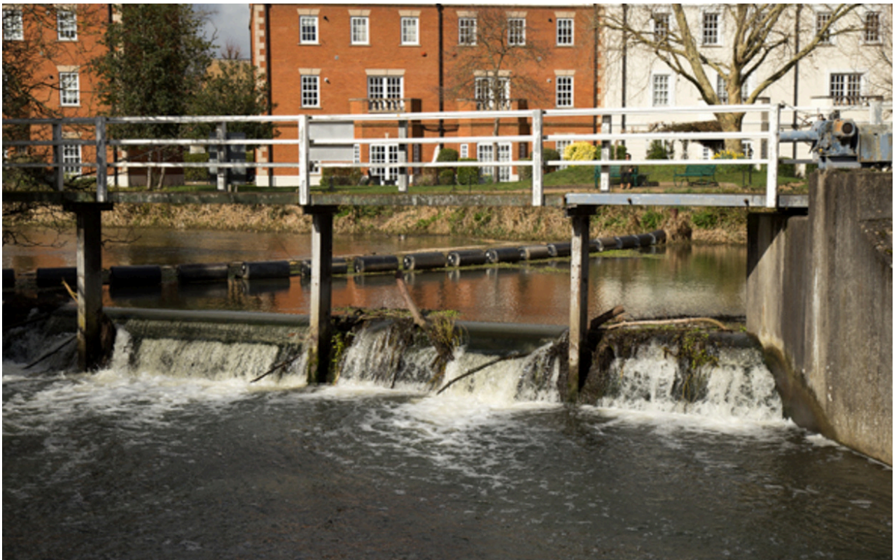
Zenith Sluice on the River Mole, which currently prevents fish passage.
