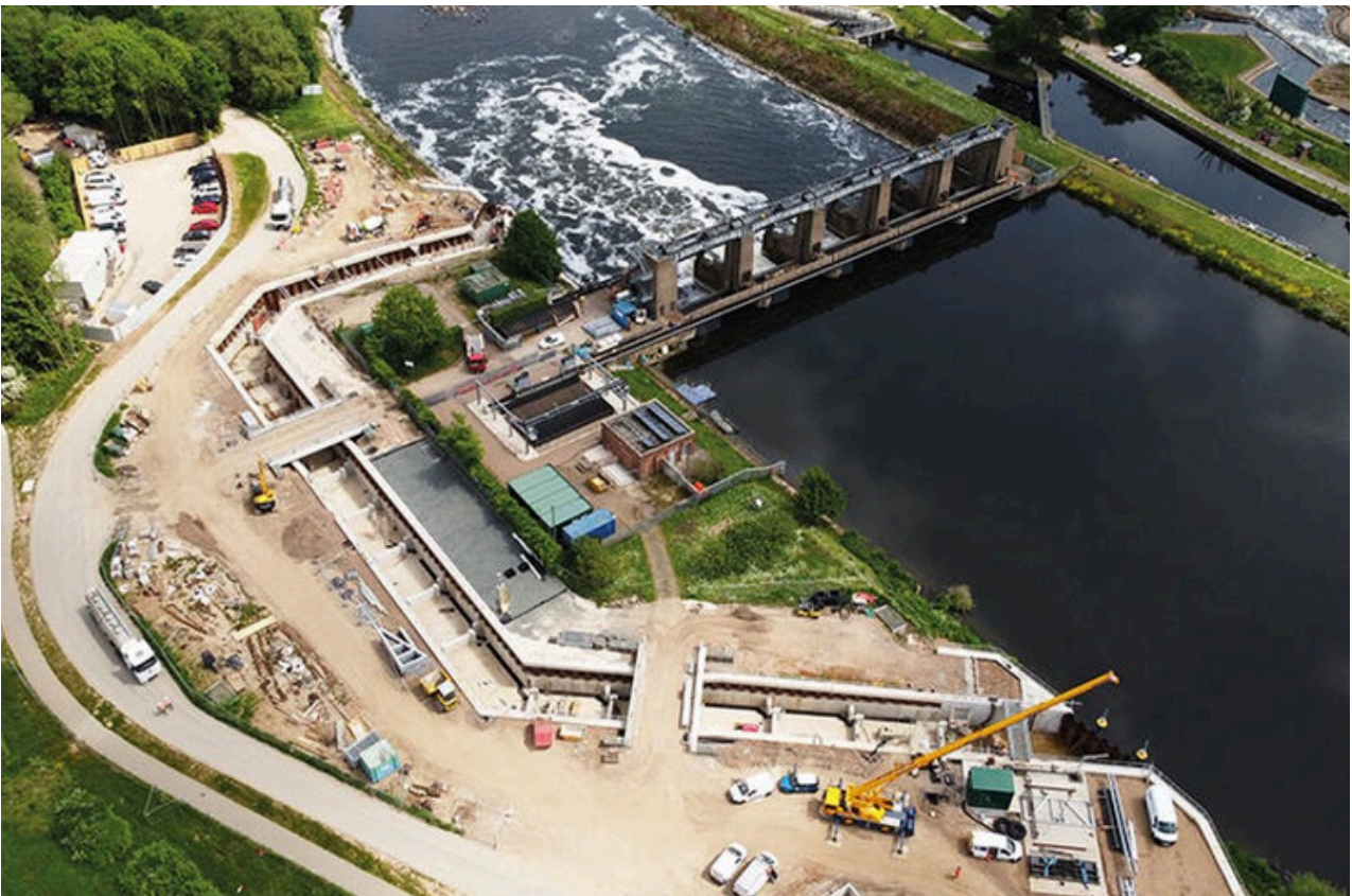
The UK's biggest fish pass was constructed at Holme Sluices on the River Trent, but other weirs remain impassable.
