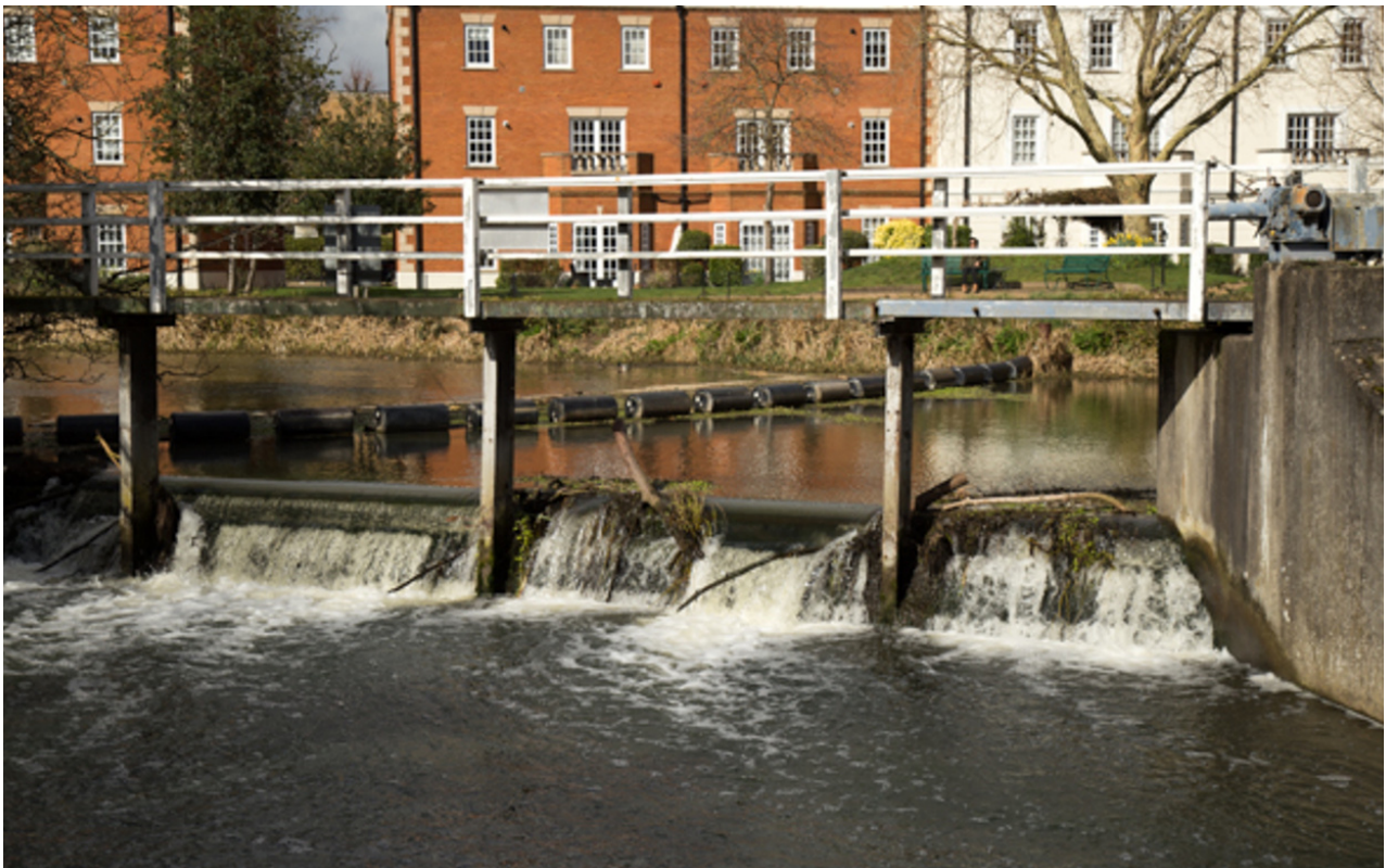
Zenith Sluice on the River Mole, which currently prevents fish passage. ©EnvironmentAgency
