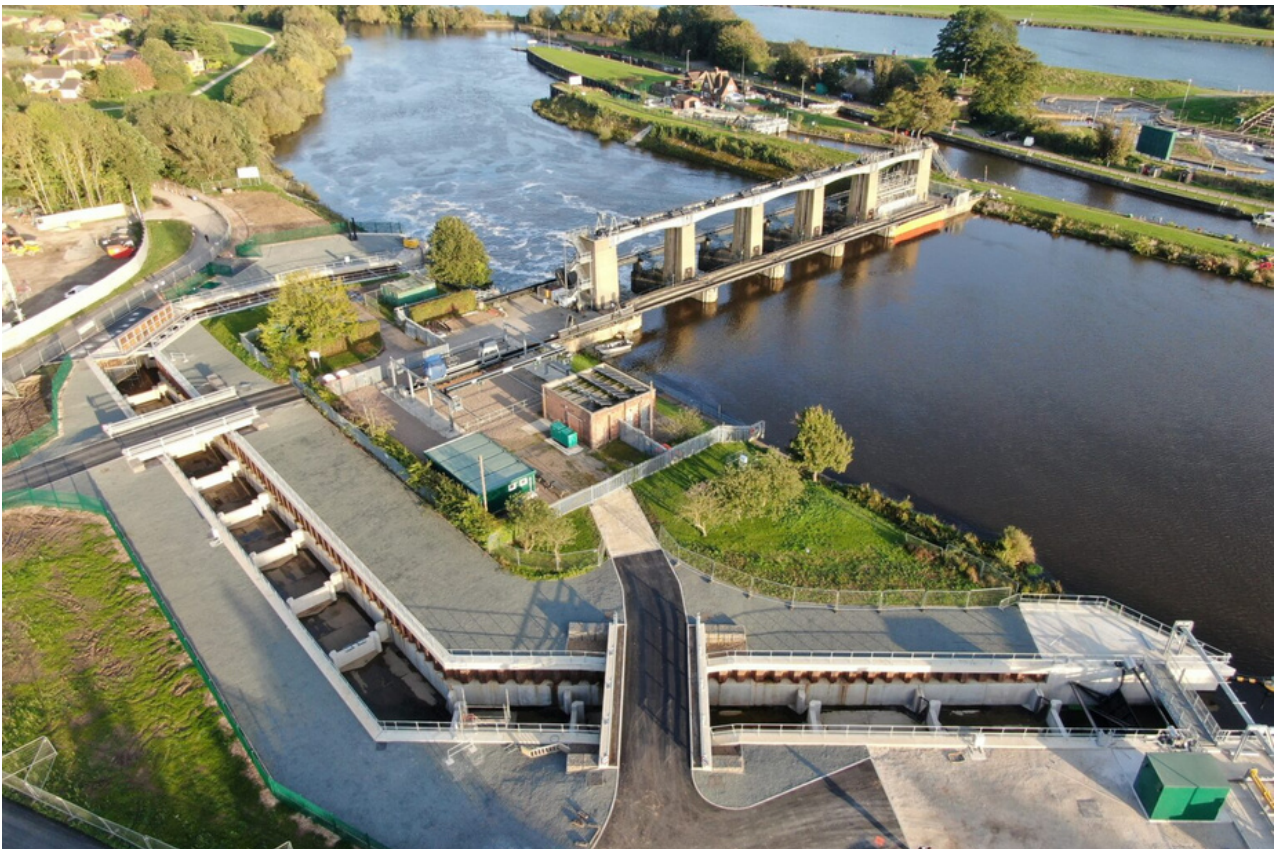
The UK's biggest fish pass was constructed at Holme Sluices on the River Trent, but other weirs remain impassable. ©EnvironmentAgency
